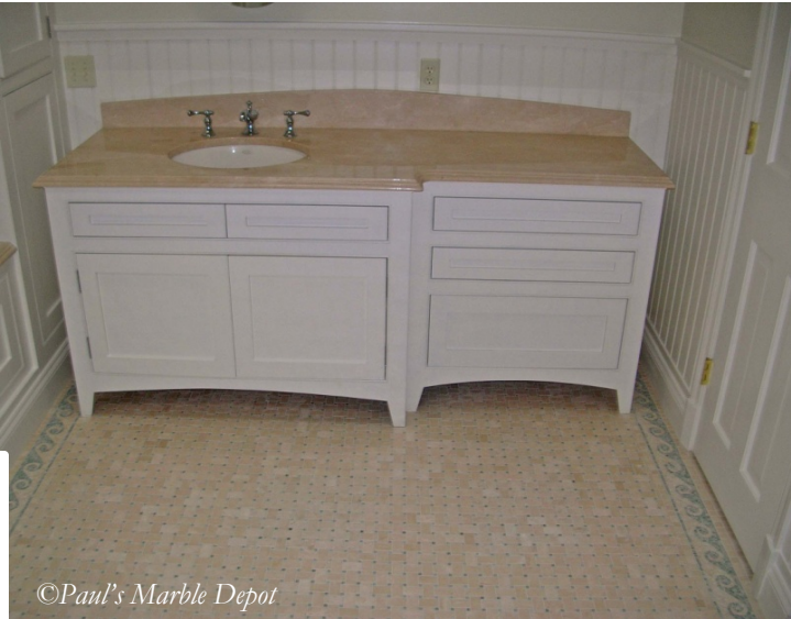
This page and Opposite: A master bathroom for a house in Pound Ridge, New York, designed by Woodsbed Design. Basket weave for flooring, 160sft, and decorative border, 80lft, was manufactured in-house, in custom colors and size. Tub deck and the two vanity tops in Crema Marfil, an inch and a quarter thick.
